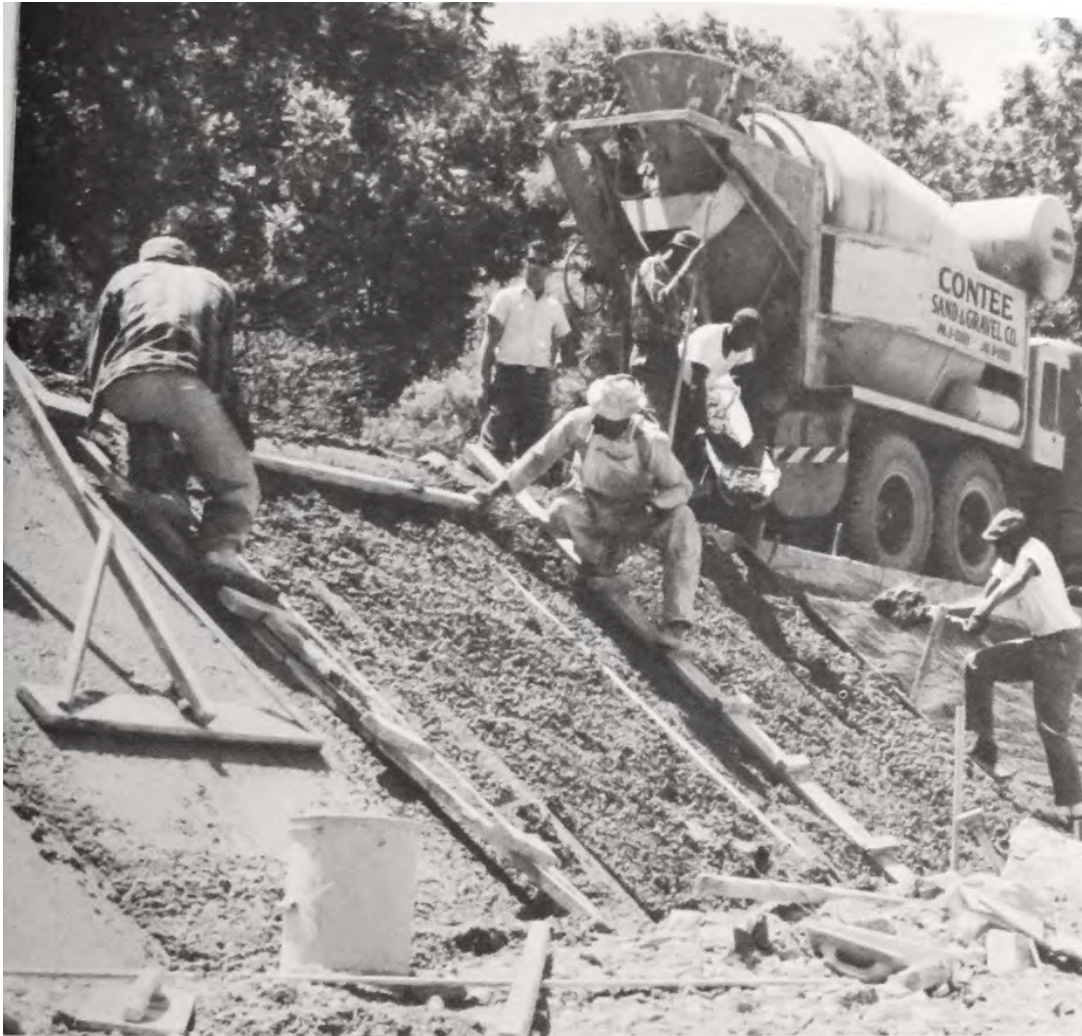
Huge channels and pipelines are designed and constructed by the WSSC to solve storm drainage problems. Workmen are shown channelizing a section of the million-dollar Willett Branch Drain in Montgomery County.
