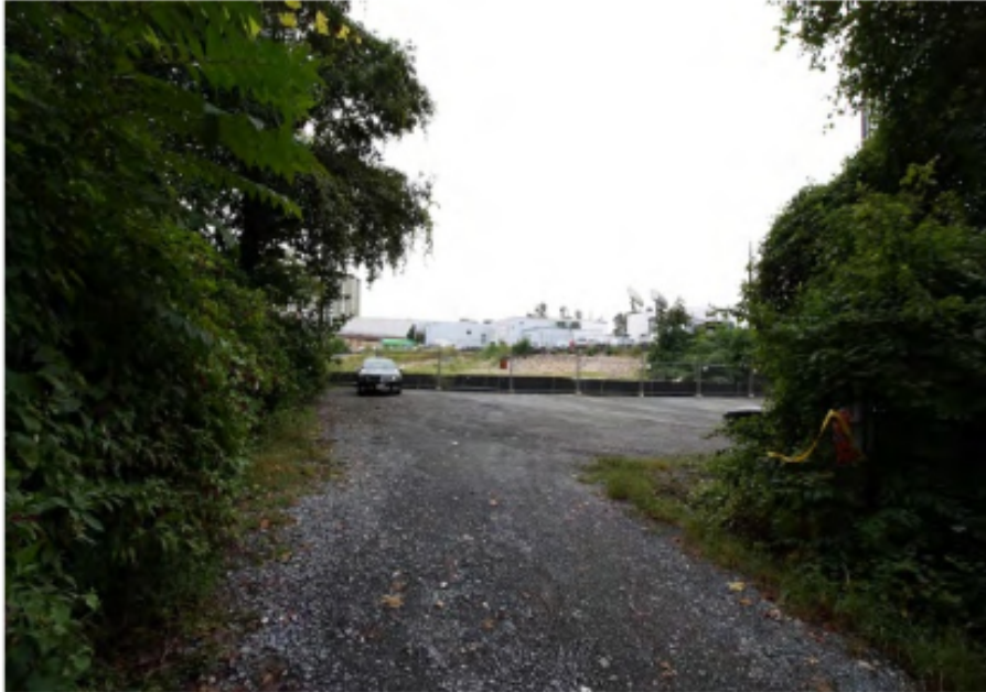
Figure 6. River Road Moses Cemetery: Parcel 177 under construction, view to the north.
