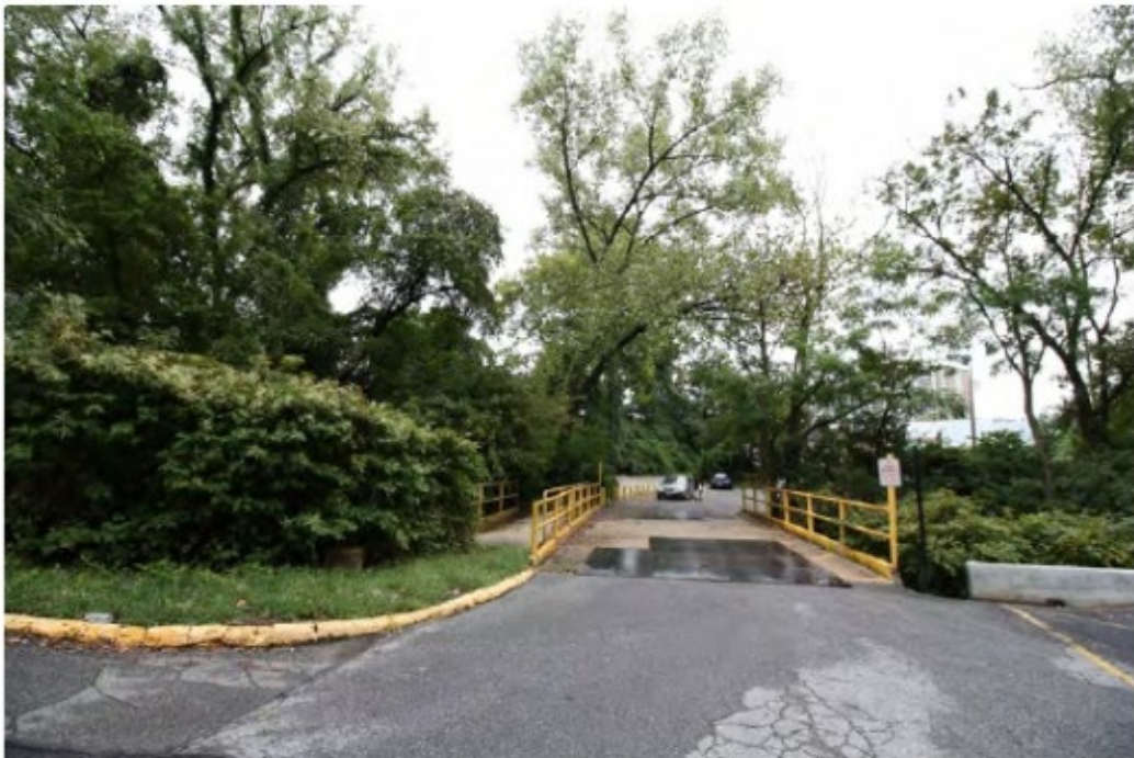
Figure 5. River Road Moses Cemetery (Parcel 175): Bridge across Willett Branch, view to the north.
