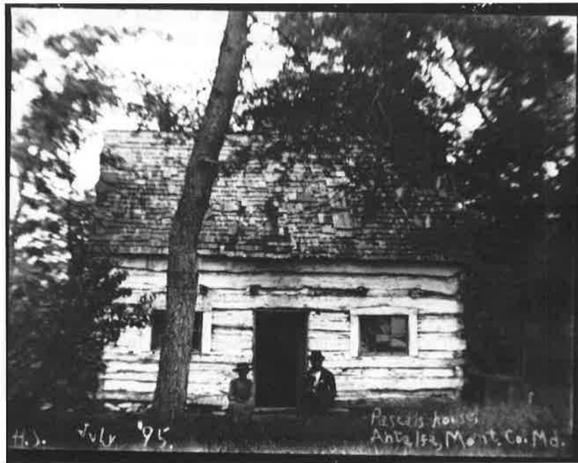
Figure 21. House believed to be where Pascal Botts lived on the Solyom property. Photo courtesy of Steve Lane.
